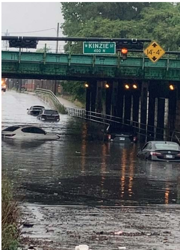
Figure 13: Vehicles stranded in flooded viaduct
