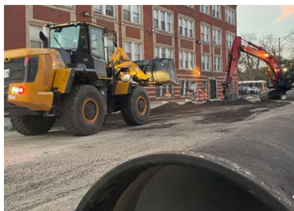
Figure 21: Construction of Sewer Lines
