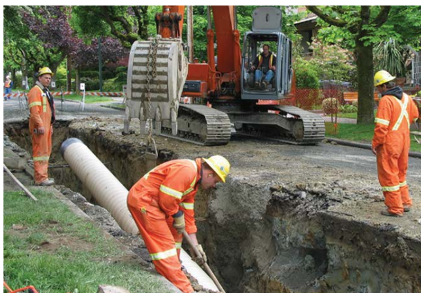
Figure 20: Excavation of Sewer Lines
